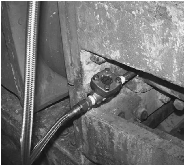
FIGURE 14.4 Thick stock pump improved Check Valves.
