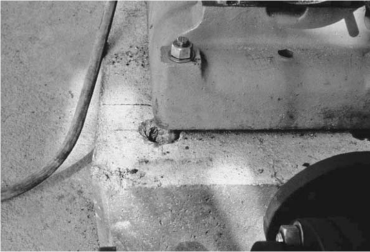
FIGURE 7.3 Loose anchor bolts on equipment base.
