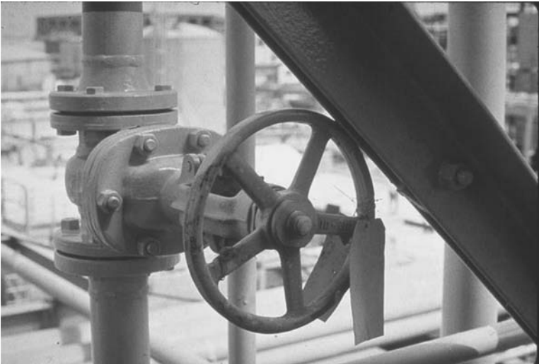
FIGURE 7.2 Pinch point created by equipment layout.
