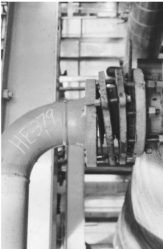
FIGURE 7.4 Pipe misalignment.
