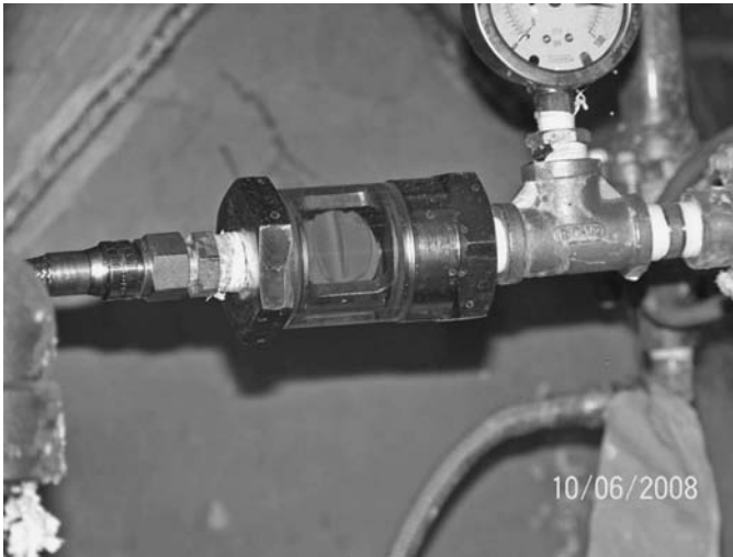
FIGURE 14.3 Thick stock pump Visual Flow Indicators.
