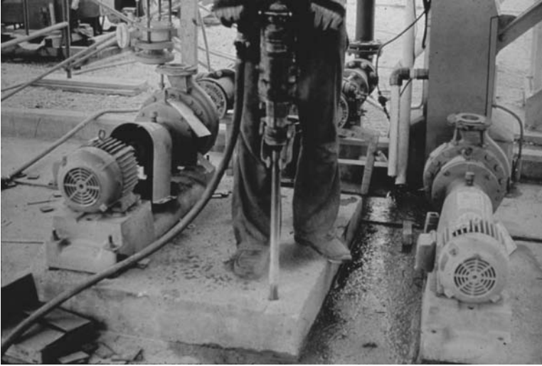
FIGURE 7.1 Jackhammer used on base of new pump.
